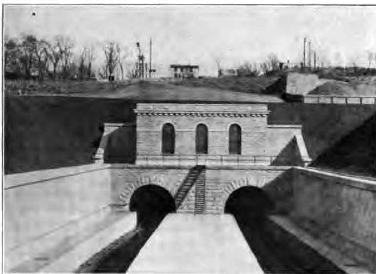
THE HACKENSACK PORTALS OF THE PENNSYLVANIA'S GREAT TUNNELS UNDER NEW YORK CITY
